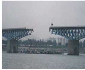
Sung-Soo Grand Bridge in Seoul: one span fell into the river as a result of breakup of the linkage pins due to heavy traffic, 1994
