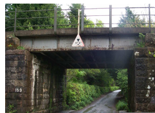
Photo of the bridge
